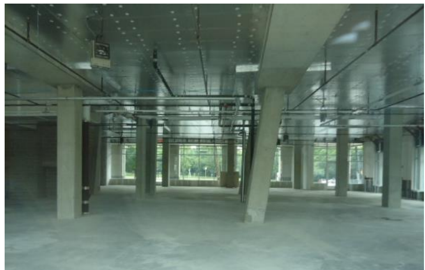
Figure 9: Sloped Columns in Retail Space
