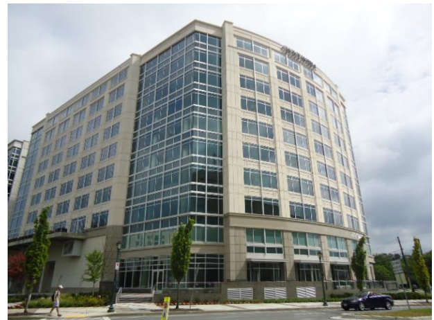
Figure 1: South West Corner – by JMV
